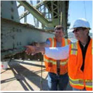
The 90 year old Hood River Interstate Bridge requires constant maintenance
