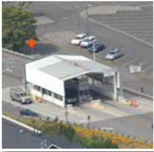
Hood River Interstate Bridge Toll Booth
