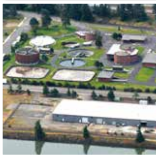
Hood River sewage treatment plant
