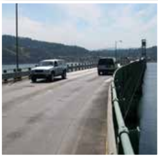
The north approach onto the Hood River Interstate Bridge
