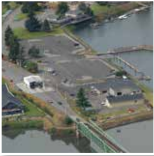
Hood River Intersate Bridge toll booth, Marina boat launch and Port offices
