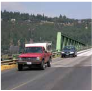
Vehicles arriving in Oregon on the south side of the Hood River Interstate Bridge
