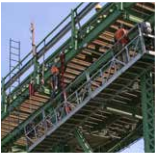
Hood River Bridge maintenance
