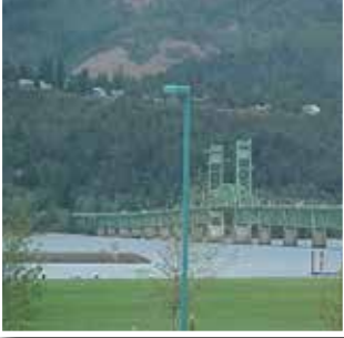
The Hood River Interstate Bridge as seen from the marina green
